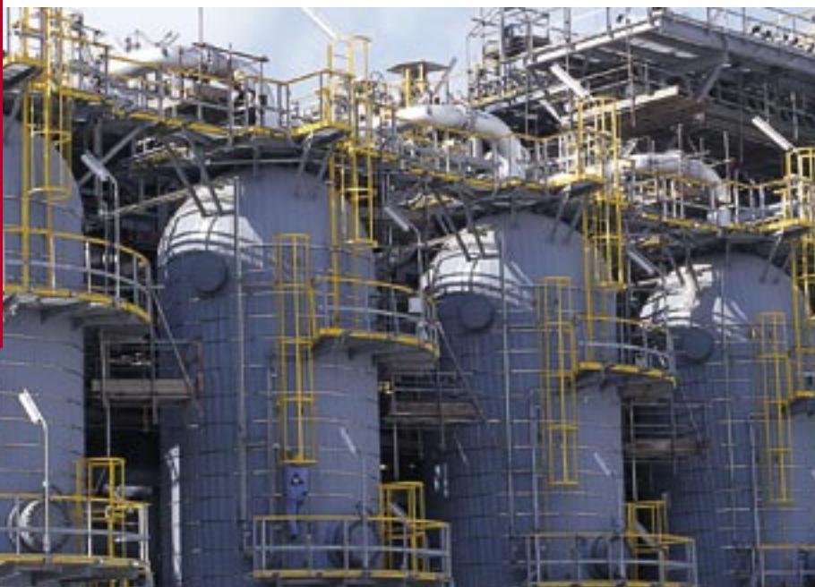
State-of-the-art LNG trains are designed to expand production of Qatar's North Field.
