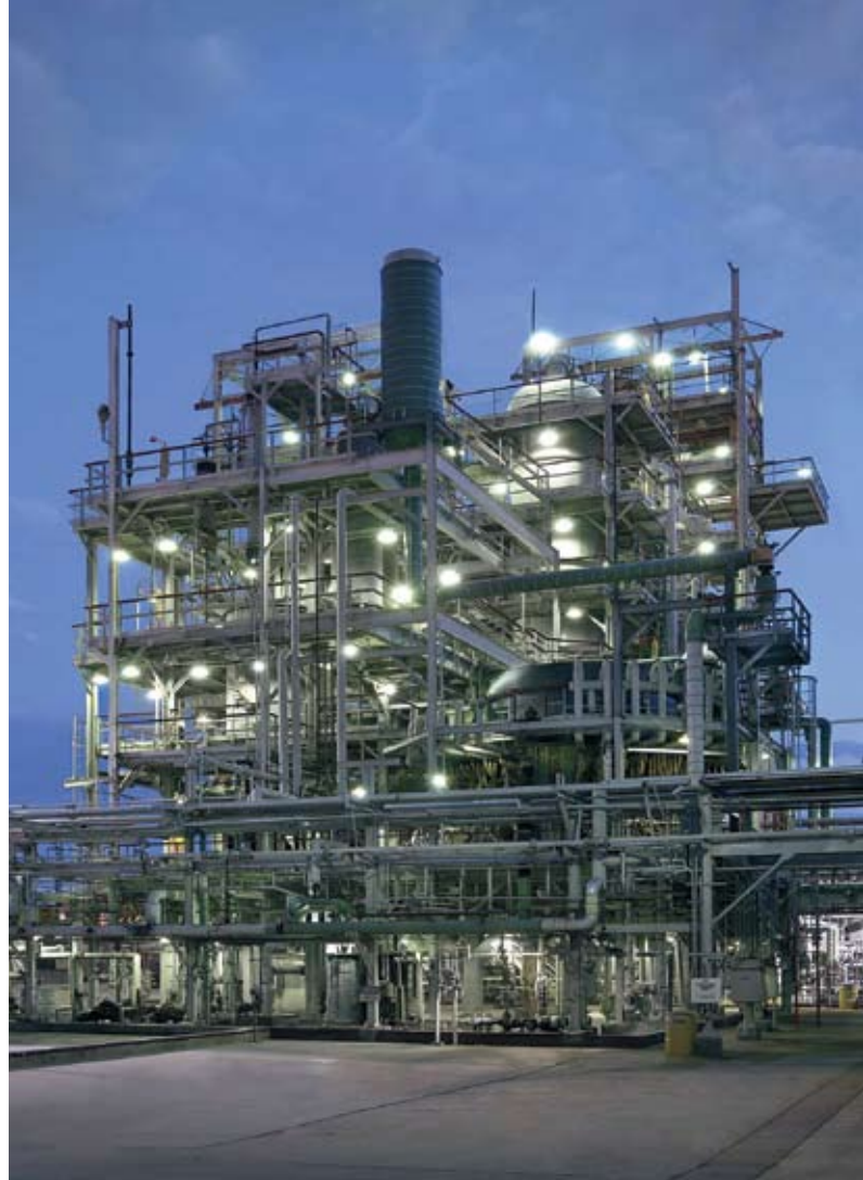
ExxonMobil Chemical's Baton Rouge facility will boost production capacity to meet the world's growing demand for isopropyl alcohol.
