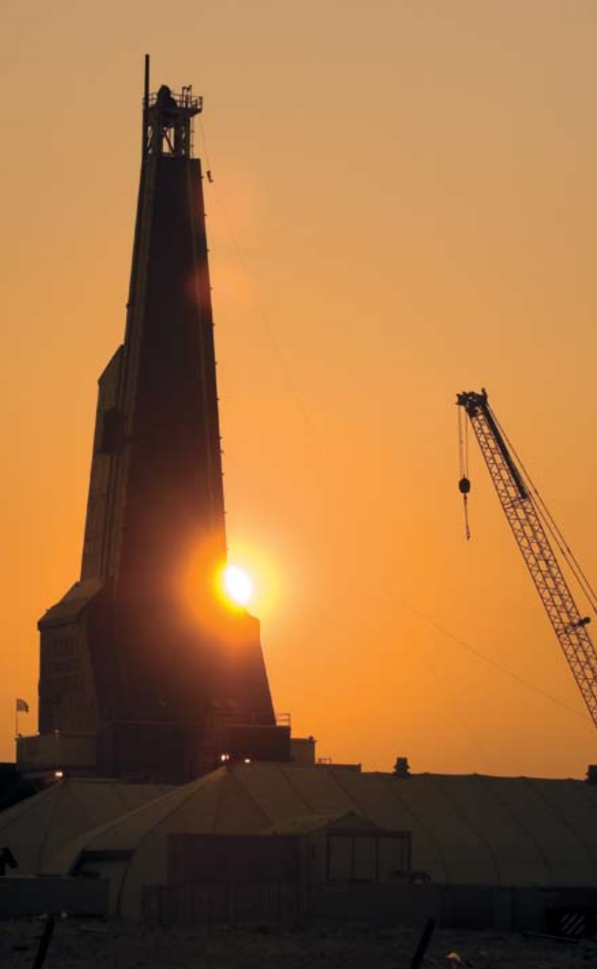
The Yastrebov rig uses extended-reach drilling that bores horizontally under the sea for six miles to reach the Chayvo field.
